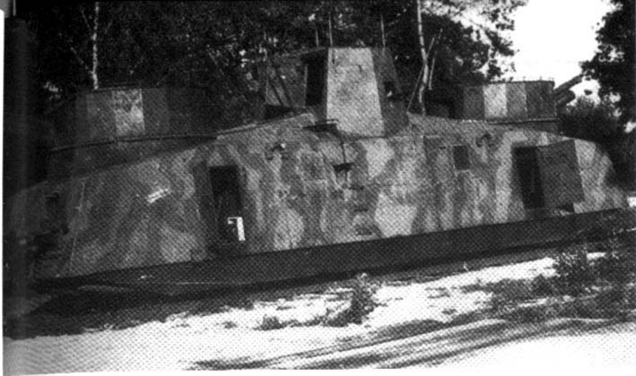
Lower right: The Panzerjäger railcars (No. 51 ff.) with Panzer IV turrets (7.5-cm KwK, long) were finished before the war ended, but they never got into service. The Americans found them as seen here at the factory in Steyr when the war ended.(LO)
