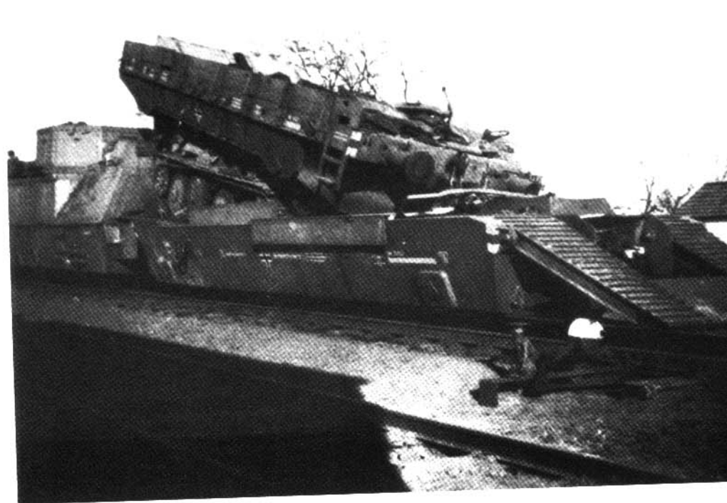
Above: On March 11, 1944 Armored Train No. 30 was rammed by an ammunition train at Lozinko (north of Nikolaiev). The pusher car was pushed up onto the tank-carrier car. Below: What remained of an armored train damaged in a fight with Russian tanks.(1 x SA, 1 x KR)
