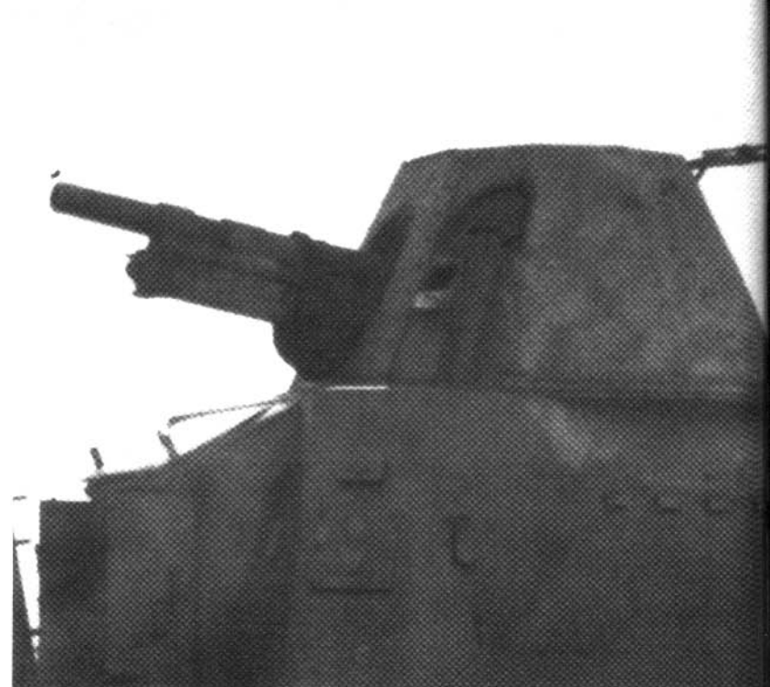
The guns of the BP 42 armored train. At left is the 7.62-cm 295/1(r) field cannon, the Russian M 02/30 with the shorter L/30 barrel (Vo 635 m/sec, maximum range 12 km); at right the Skoda 14/19 10-cm light field howitzer, from captured Polish and probably also from Czech material (Vo 395 m/sec, maximum range 9.8 km).(BA)
