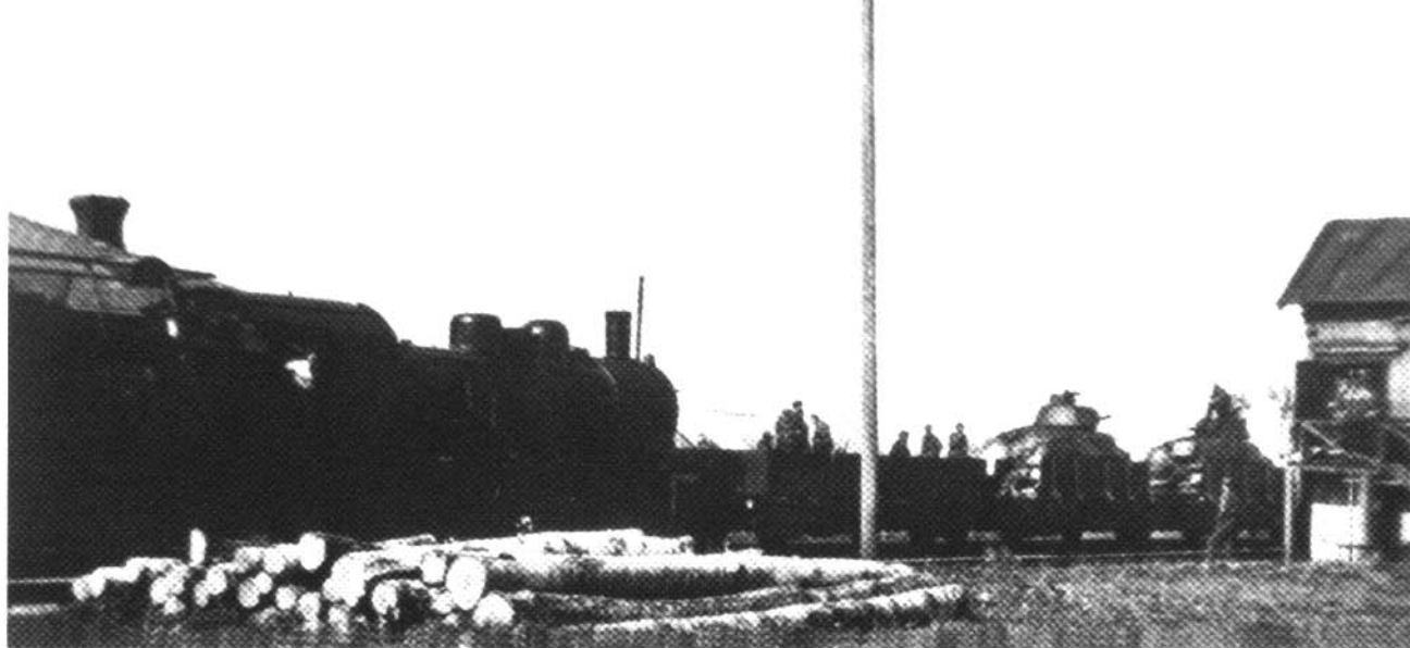
The auxiliary broad-gauge armored trains prepared for the Russian campaign, that consisted only of tank-carrying cars with removable captured French Somua S 35 tanks, infantry cars open at the top, and a Series 57 locomotive with only its cab armored. Above is Armored Train No. 28 (Army Group Center).(1 x SA, 1 x BA)
