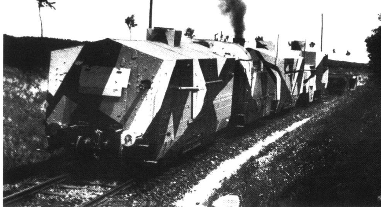
Above: Czech armored train (built 1919); the material of the three armored trains of this type was utilized as of 1940 in German armored trains 23 to 25.
